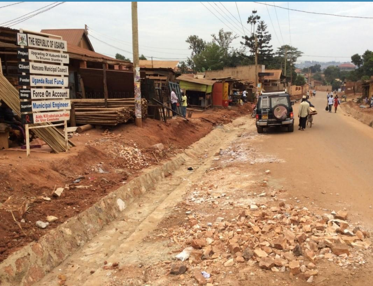
Rainwater Drainage in Kampala
